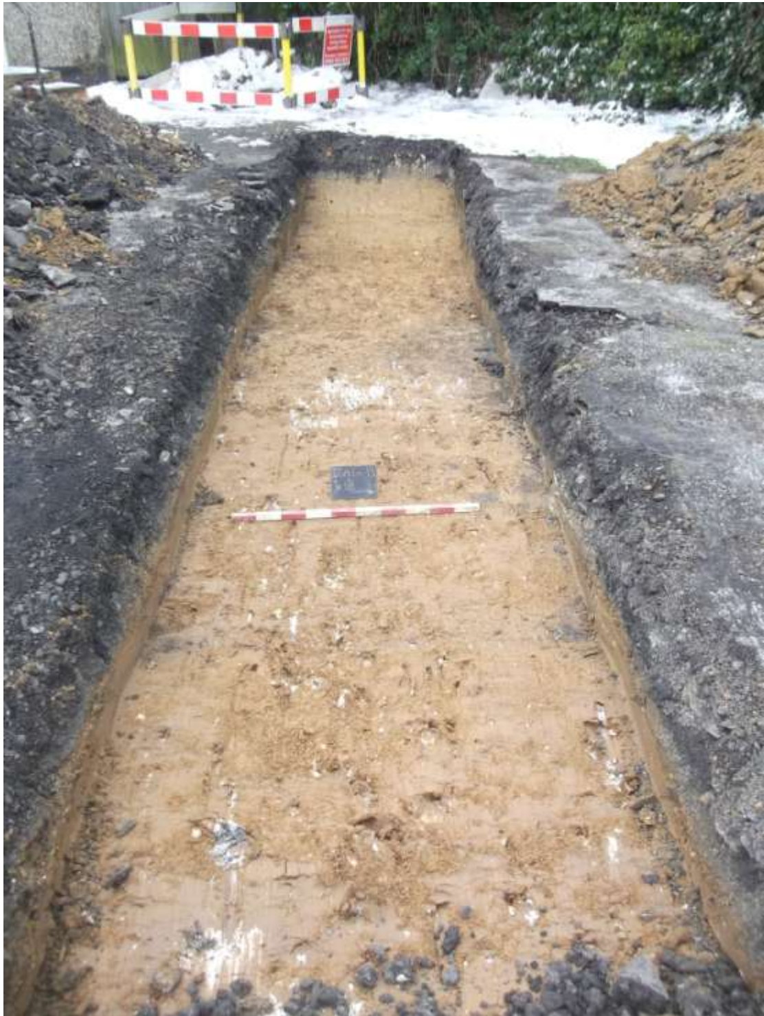
Plate 5. Trench 1b looking north-west
